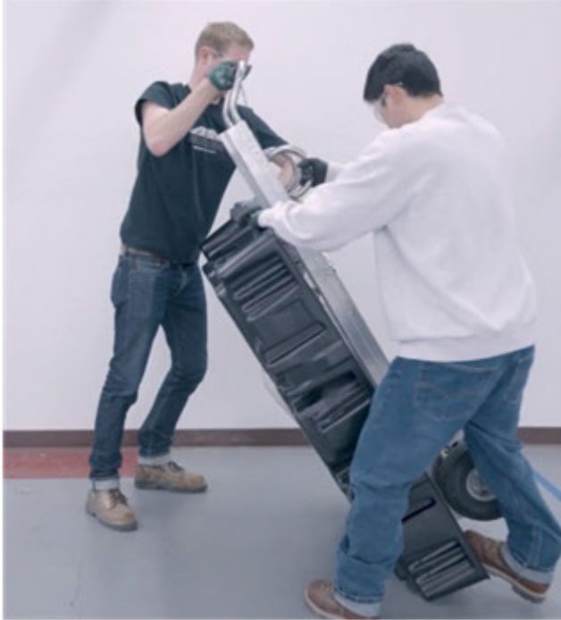
Figure 5. Tilting the Dolly and Powerwall Up with the Brake Engaged
