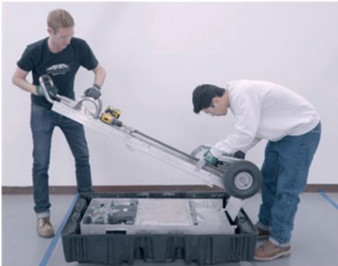
Figure 1. Lifting Plate in Gap Below Powerwall
