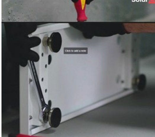
Figure 5: Floor Stand Leveling
